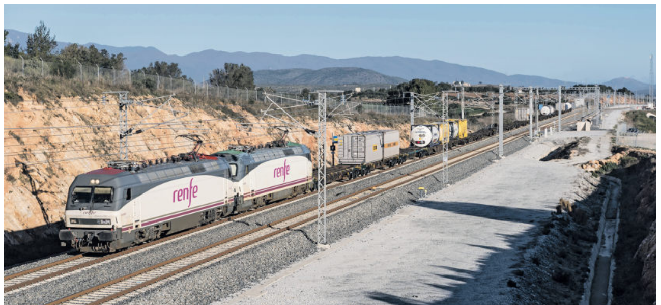
A train through the first UIC corridor connecting the Iberian Peninsula with Europe.
