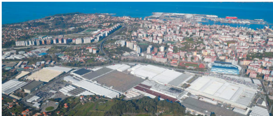
Close-up image of the Balaídos industrial estate (Vigo), which is home to PSA's automotive factory, and where it plans to produce hydrogen for logistics use / CZFV
