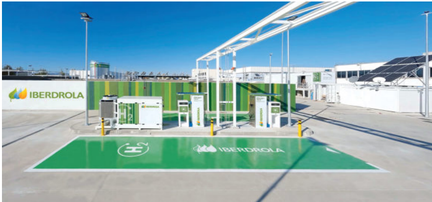
Green hydrogen refuelling station at the Zona Franca Consortium in Barcelona.
