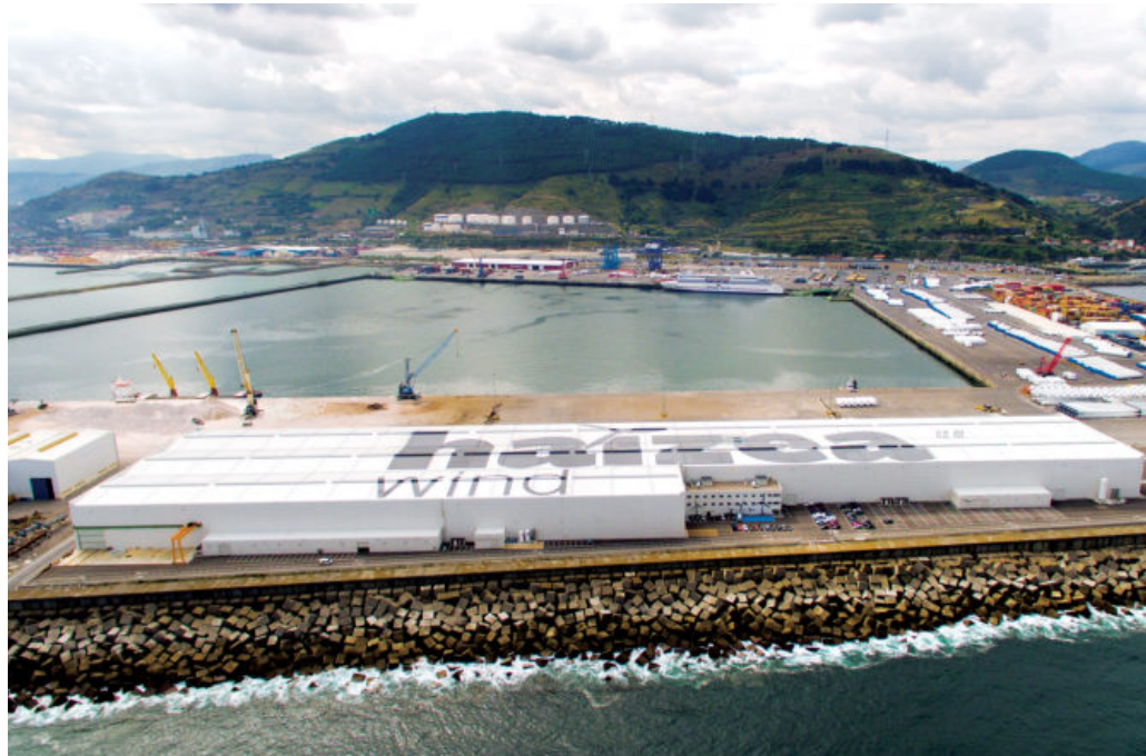
Image of the Haizea Wind facilities in the port of Bilbao.
