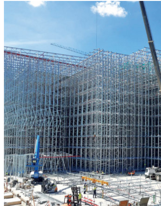
Virto refrigerated warehouse under construction in Funes (Navarra).
