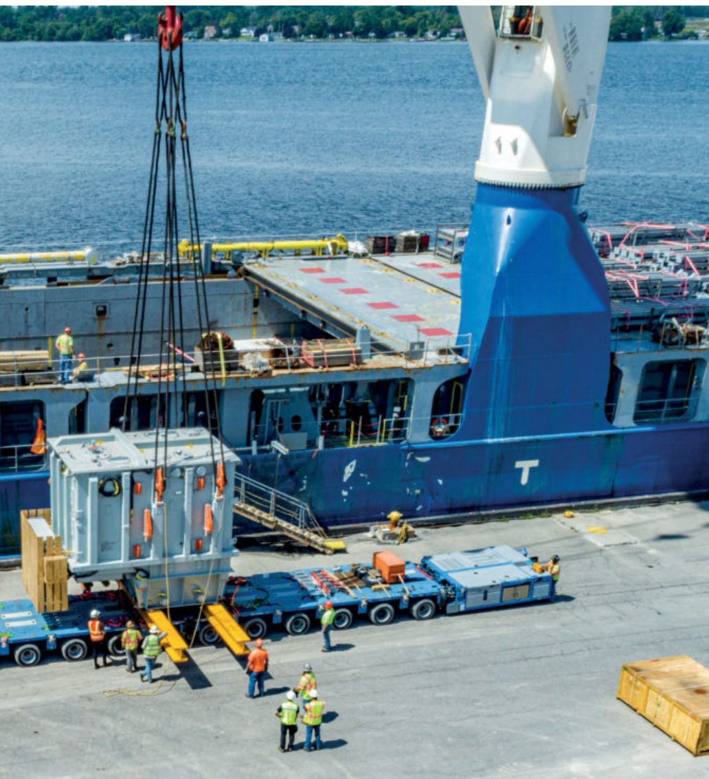
Loading of a transformer in the United States.
