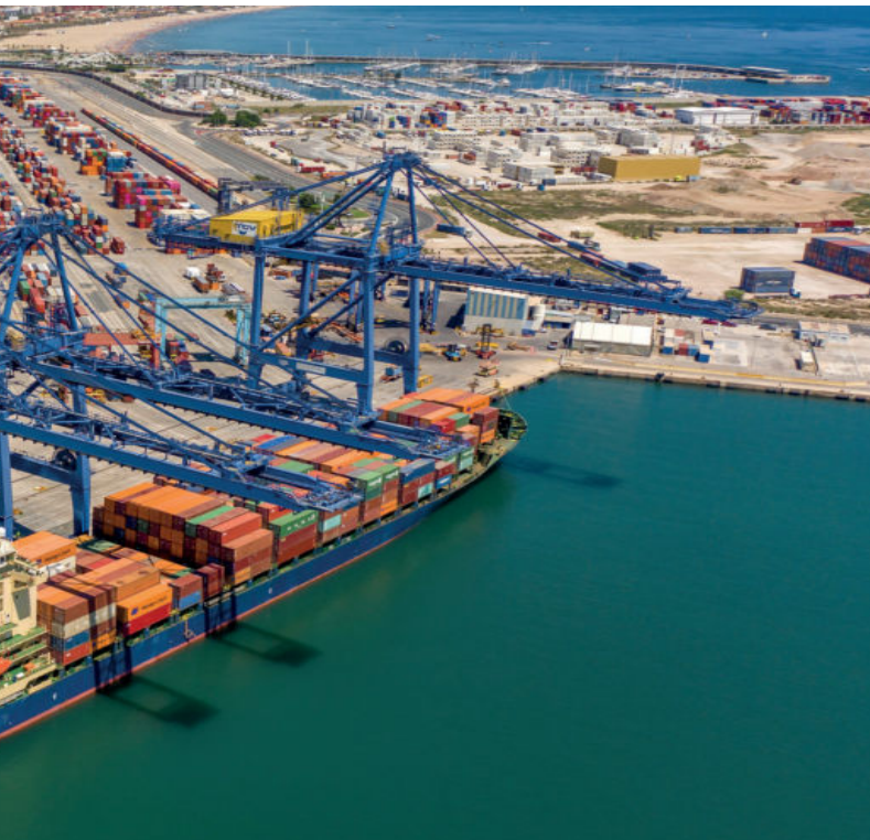
Technology can already detect an accident involving a crane while it can still be avoided.
